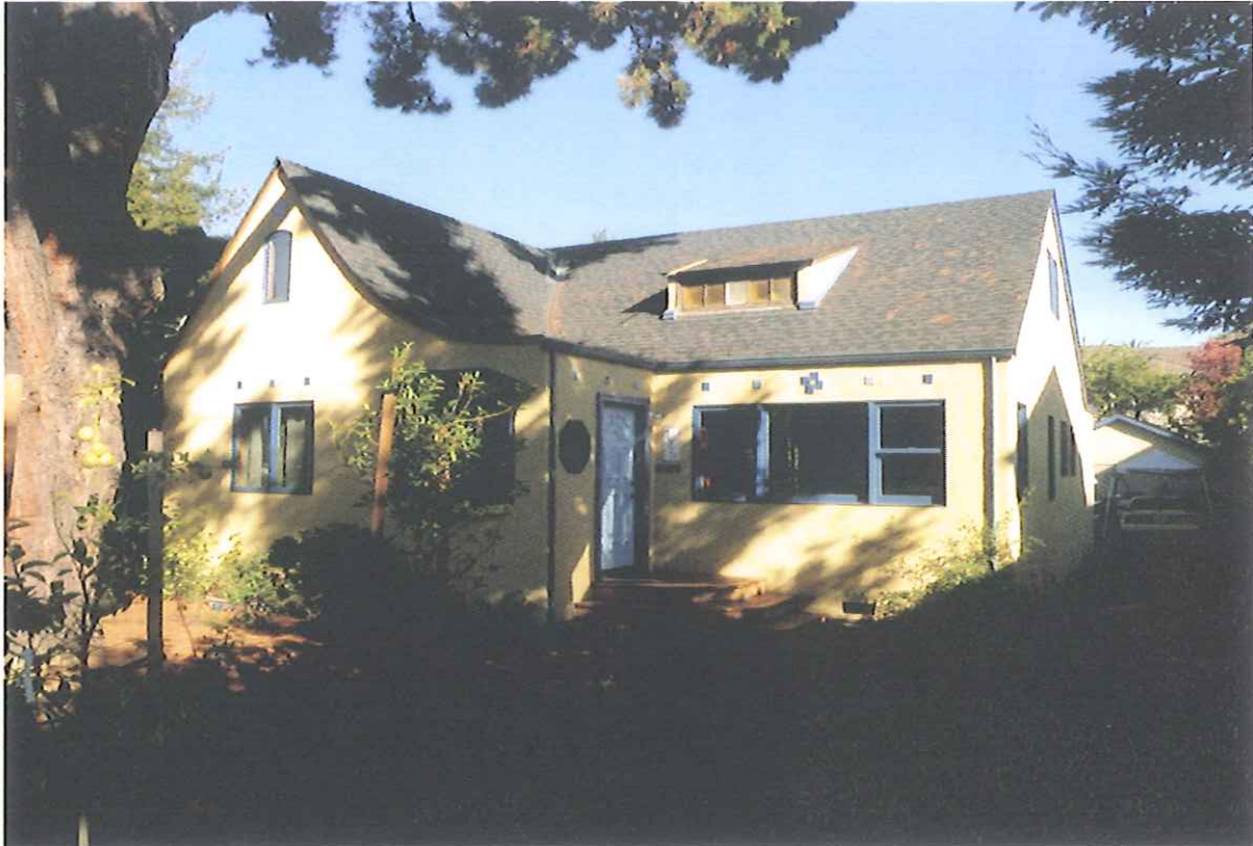
Date Taken: 10/19/2011 Photo ID: MGVD001 10-19-11 - 125 Front overview.
